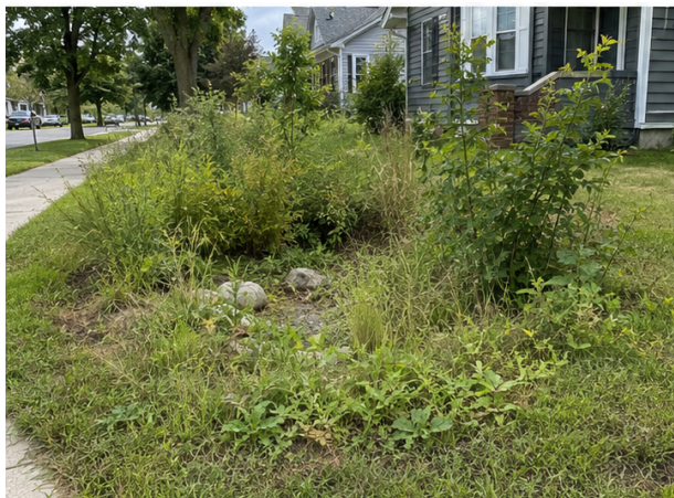
Rain garden with lost boundaries and uncontrolled growth
